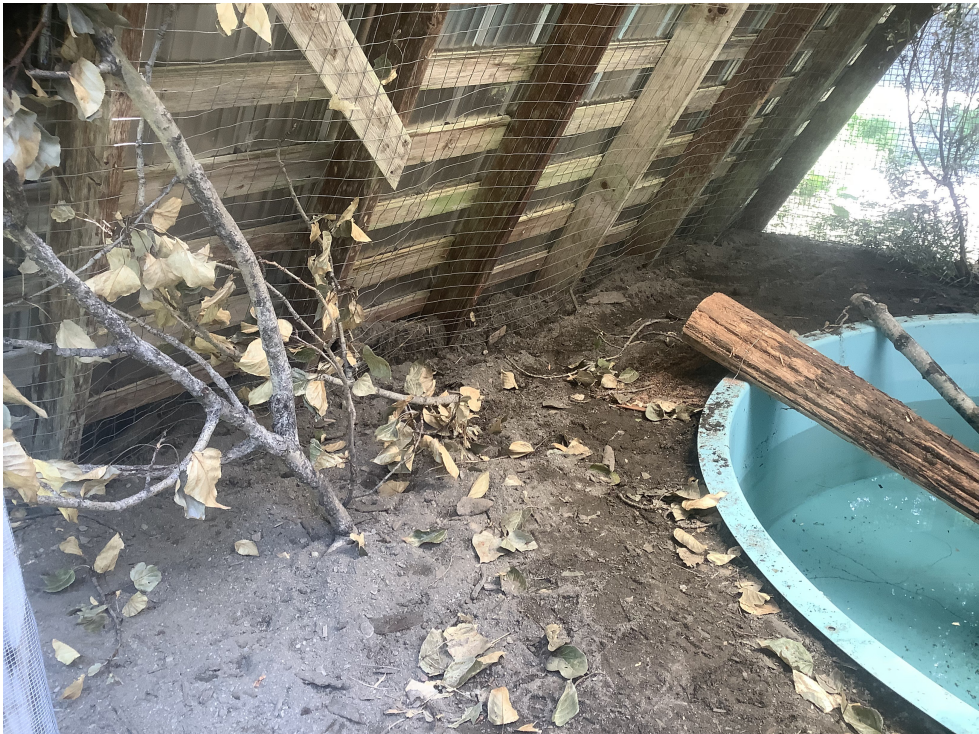
Preparing the quarantine hut. Wire under ~ 50 cm dirt and up the walls
