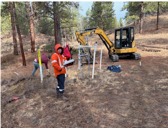
Photo 9: FortisBC overseeing post removal and installation alongside its main pipeline and farm tap junction, Nov. 2025
