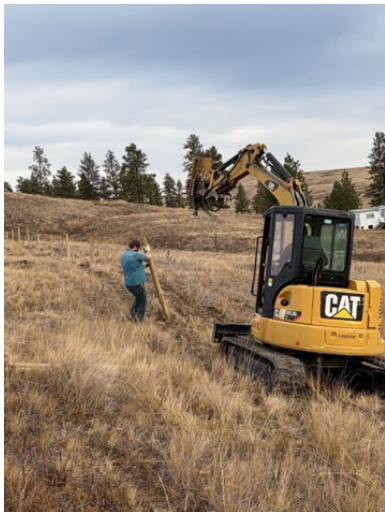
Photo 11: Darkside Fencing Ltd. installing new posts for the replacement fence, Nov. 2024
