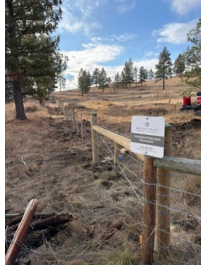
Photo 14: Same location after new fence construction, Nov. 2024
