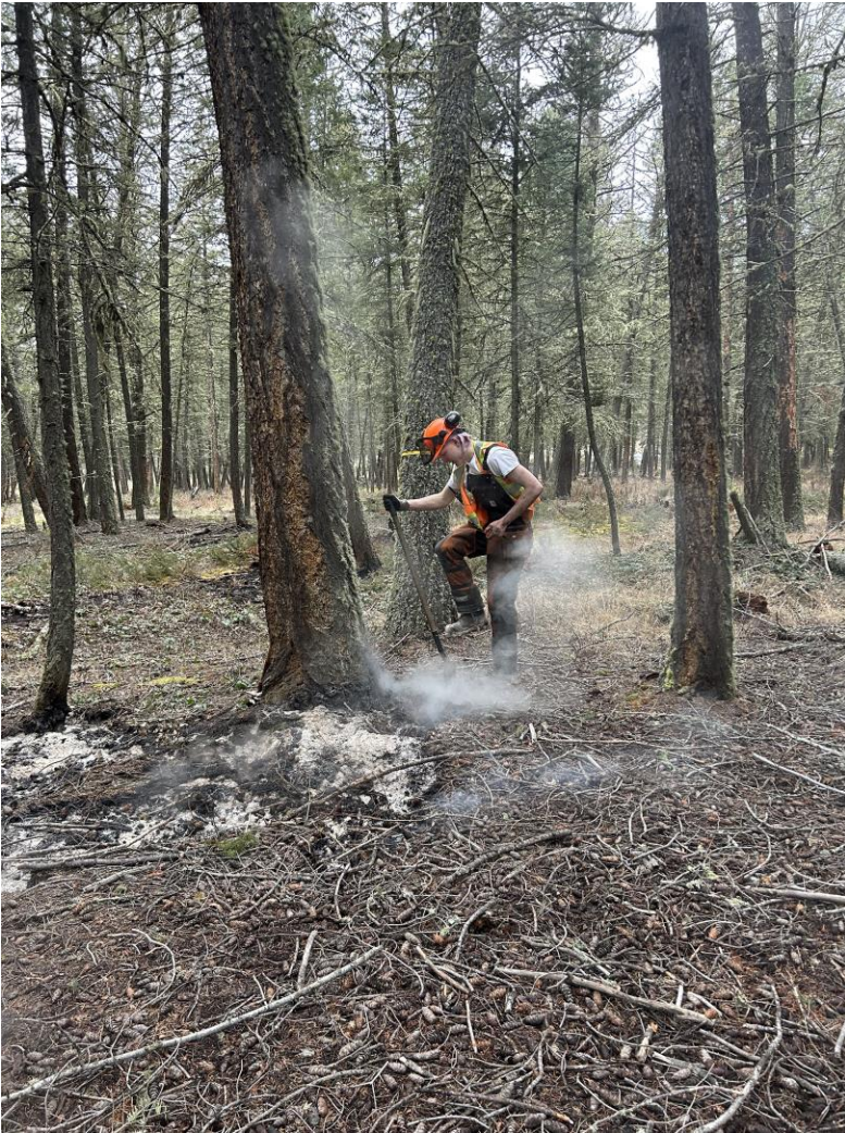
Photo 1 : A contractor works to extinguish a hotspot following pile-burning at Lot 48, as part of forest thinning treatments and prescribed burn preparations.
