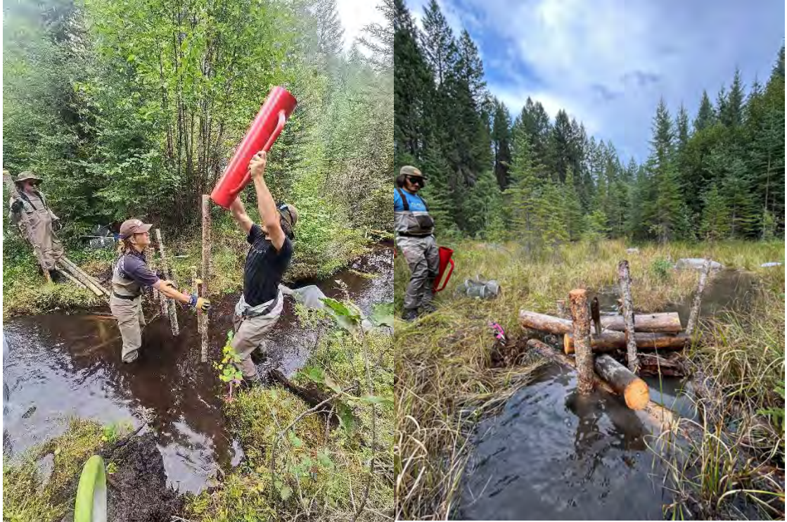
Figure 67: Pounding posts into the Limbo stream for BDA structure; PAL post-construction.
