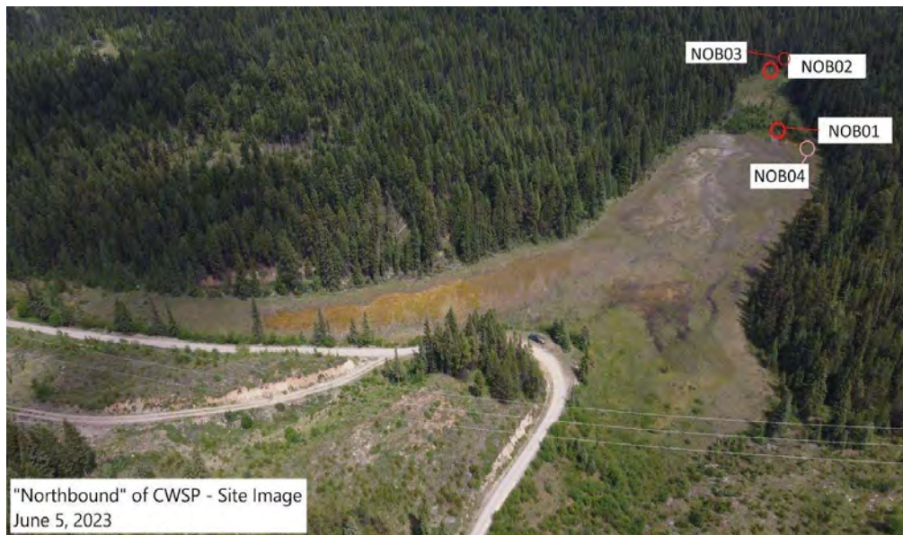
Figure 46. Drone photograph showing the locations of the proposed structures within CWSP Site "Northbound".
