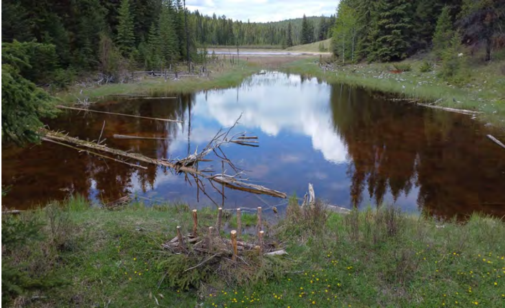
Figure 25. Upstream BDA was constructed at Beaver Channels in September 2024, showing water being held by BDA in May 2025. This area directly behind the BDA was not flooded in May 2024.
