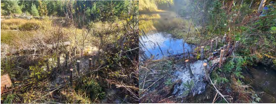
Figure 15. Photographs of the two Beaver Dam Analogues (BDAs) constructed in this wetland in September 2024. Left: Downstream BDA. Right: Upstream BDA.
