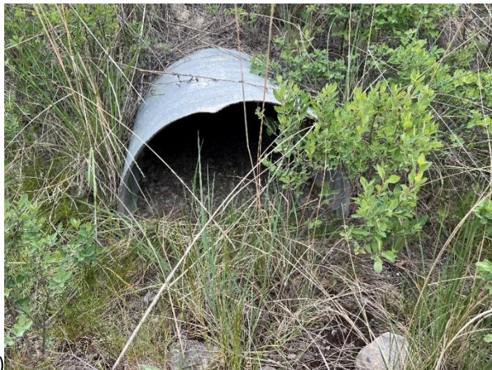
Figure 10. Culvert assessment at different types of culverts that were all assessed with high prioritization; a) large 1800 mm diameter culvert, b) small elevated culvert above a pool, c) 600 mm culvert partially blocked with substrate.
