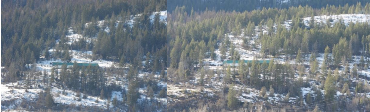
Figure 6 Pre-treatment (left – Feb 7, 2025) and post-treatment (right – Feb 24, 2026) views of slope and CVWMA Administration Office building.
