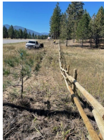
Photo 25: Job 3 during construction, September 2024
