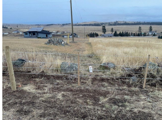
Photo 13: Job 1a after construction, November 2024
