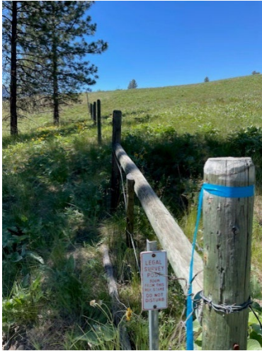
Photo 18: Job 2 fence conditions prior to removal, June 2024
