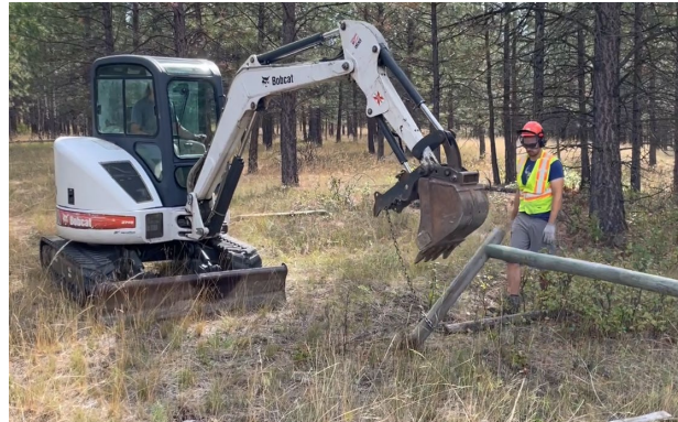
Photo 21: Job 2 required an excavator to remove posts & braces
