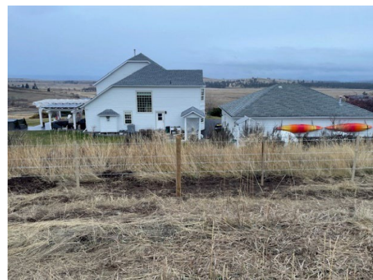
Photo 11: At times, Job 1a & 1b required access through adjacent private acreages for fence construction
