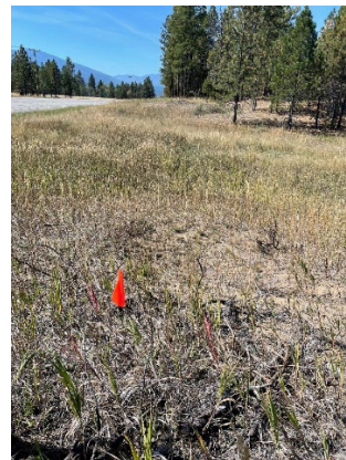
Photo 9: Pin flags show the location of buried utilities near NTBC Job 3, September 2024
