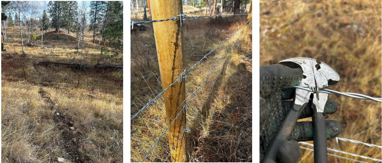
Figure 1-3: Photos of where a staple lock section was installed due to high wildlife traffic on PID 008-406-823, East Boundary, NCC
