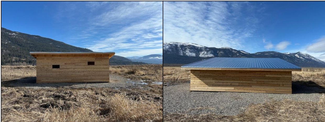
Figure 4 Wooden nesting structure with metal roof, February 27, 2025.
