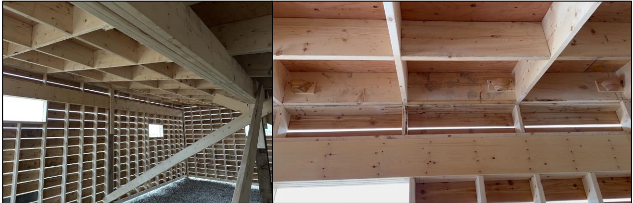
Figure 7 Internal ledges for natural nest building and wooden nest cups in ceiling compartments.
