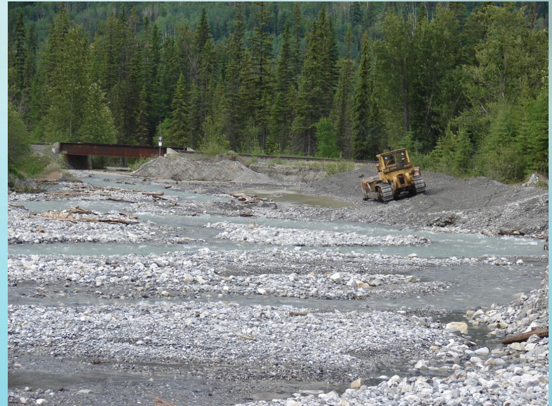
Bedload removal and tributary channelization, Horse Creek, June 2007. Photo courtesy Westslope Fisheries Ltd.
