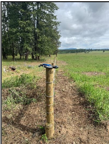
Photo 34: New fence construction underway
