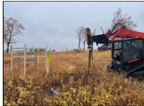
Photo 29: Installation of new fence posts in proximity to pipeline
