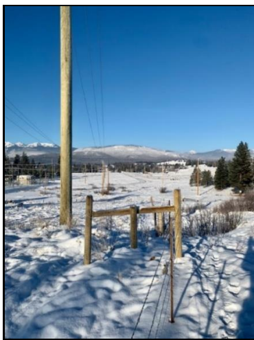
Photo 23: Fence build/bracing with setback near BC Hydro infrastructure.
