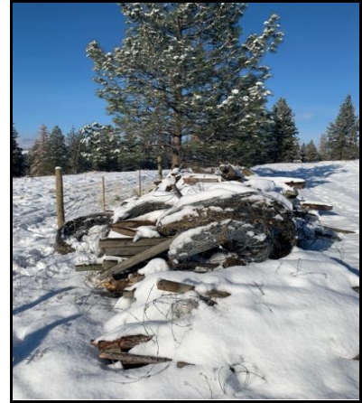
Photo 27: Fence debris ready for site removal
