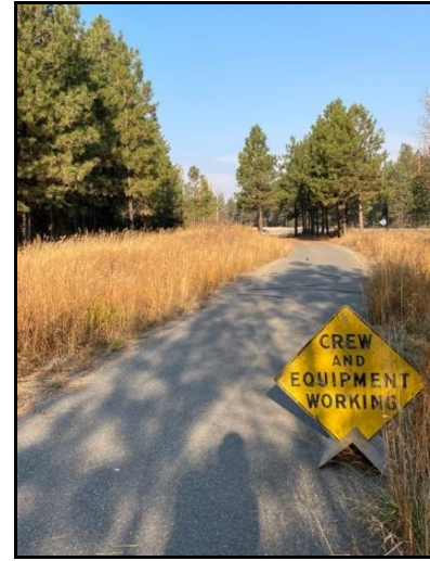
Photo 31: Required signage posted in the vicinity of work along Rails to Trails
