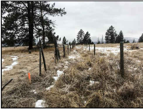
Photo 19: Double fences created a wildlife hazard, fence on the left was removed under this project.
