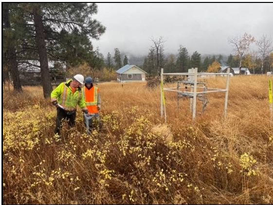
Photo 28: FortisBC staff locating pipeline prior to work
