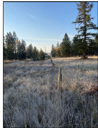
Photo 18: After repair photo on October 30, 2022
