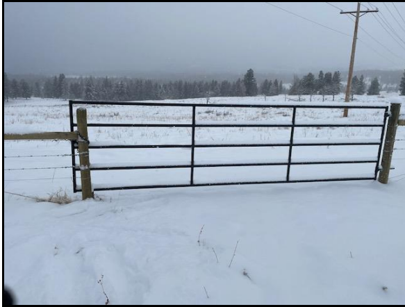
Photo 26: Metal gate on new fence at junction of BC Hydro access road
