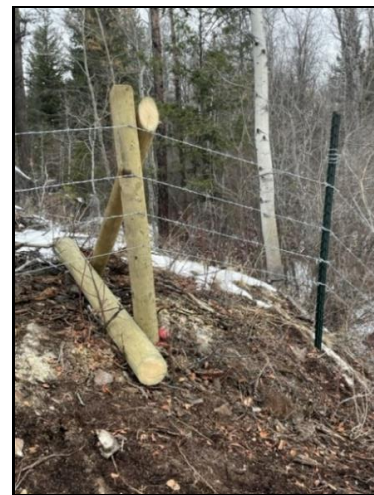
Photo 24: Bracing and T-Post on steep rocky terrain.
