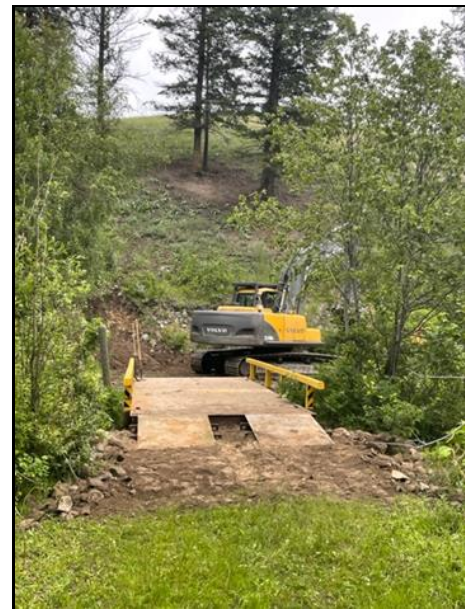
Photo 16: Installation of a temporary bridge over Luke Crk.
