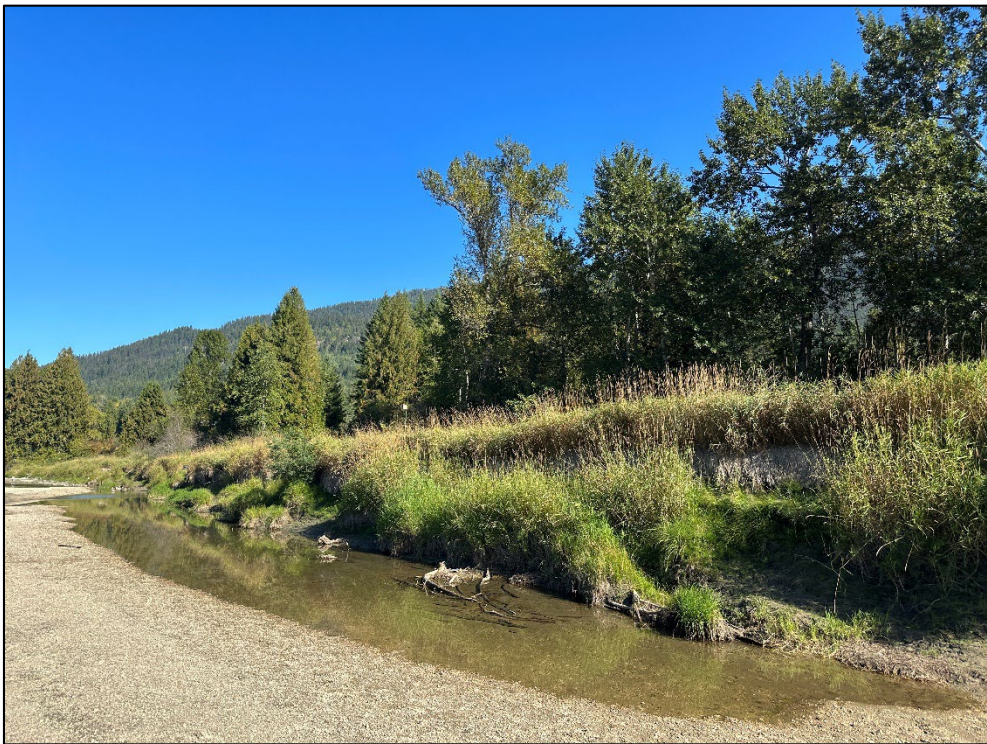
Plate 2.1-2. Severe bank erosion along the Slocan River.
