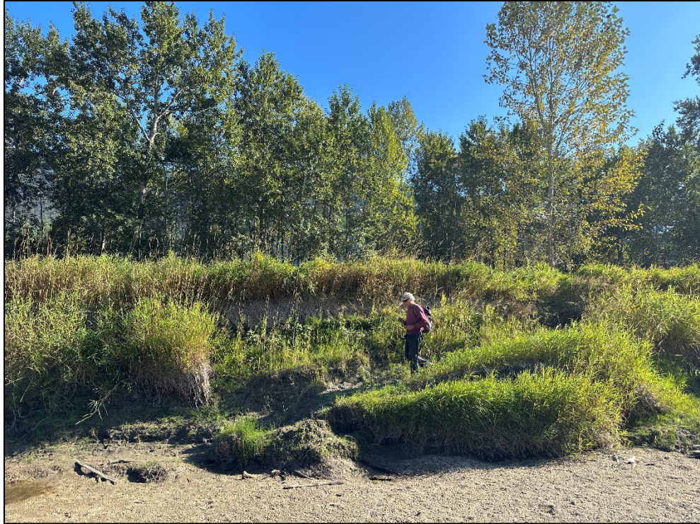
Plate 2.1-3. Example of the bank erosion exceeding 3m in height.
